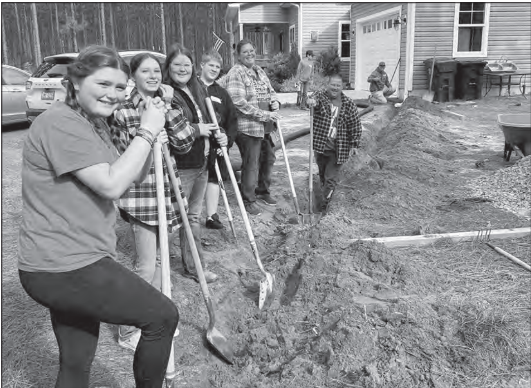
Above, members of Memorial and Dunn’s Grove churches dig a drain line during Camp Duncan’s Friends of Children (FOC) event. Below left, the Hurley family volunteered at Cameron Boys Camp’s (CBC) FOC event and brought food and dry goods as part of the Food Roundup. Below right, CBC campers proudly share their campsite and tales of life at Camp with the FOC volunteers.
